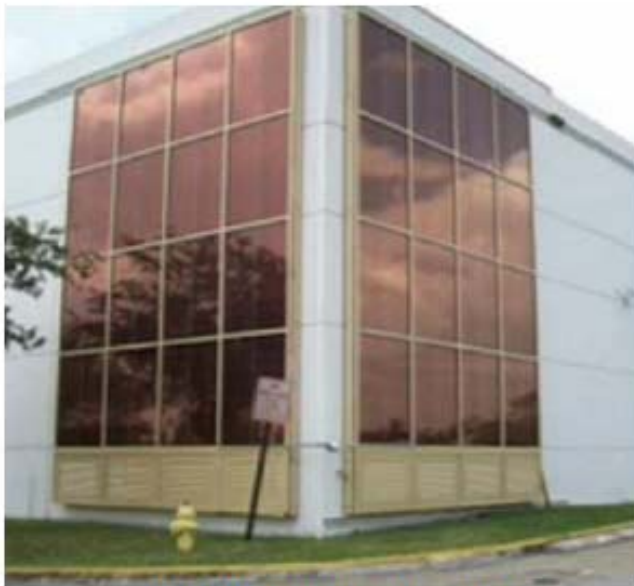
Curtain Wall Installation (Florida)
